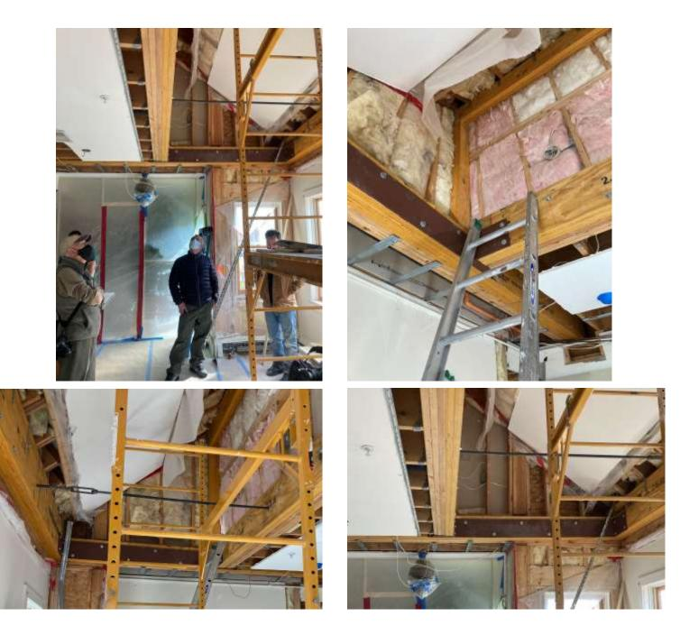
**Photo #1**: The steel plates, tie rods, and LVL reinforcing beams have all been installed at this time.
