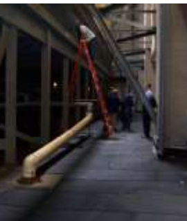
Photo #4: Existing roof beam was reinforced with new steel channels supported on new steel columns
