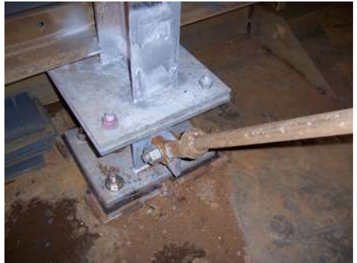
Photo #4: Existing roof beam was reinforced with new steel channels supported on new steel columns
