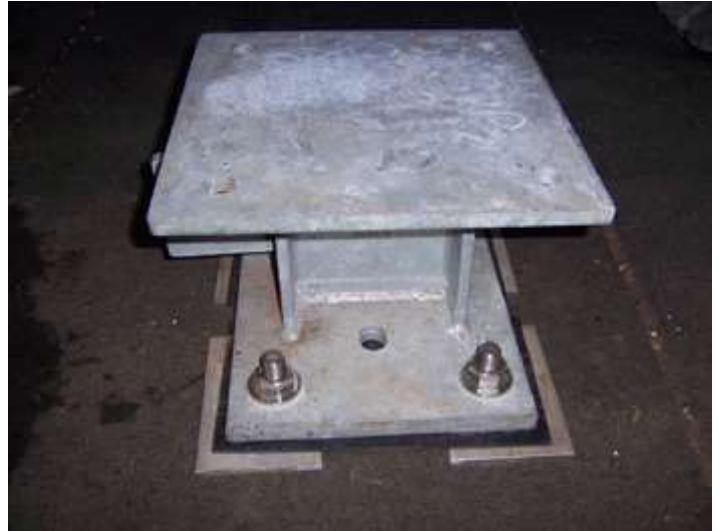
Photo #2: New Custom Fabricated Aluminum Column Base
