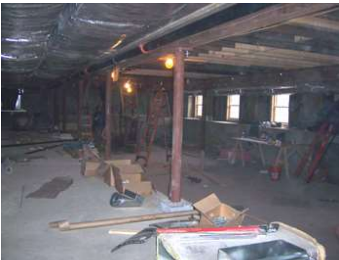
Photo #3: Basement was lowered and the walls were underpinned
