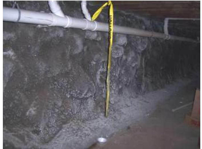
Photo #2: Basement Wall Shotcreted
