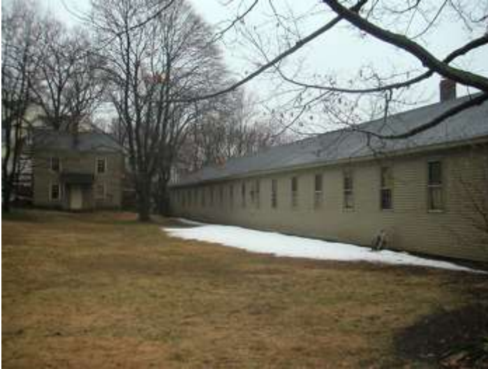
Photo #1: Building Exterior
