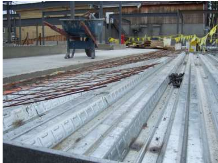
Photo #4: First floor concrete placement in progress
