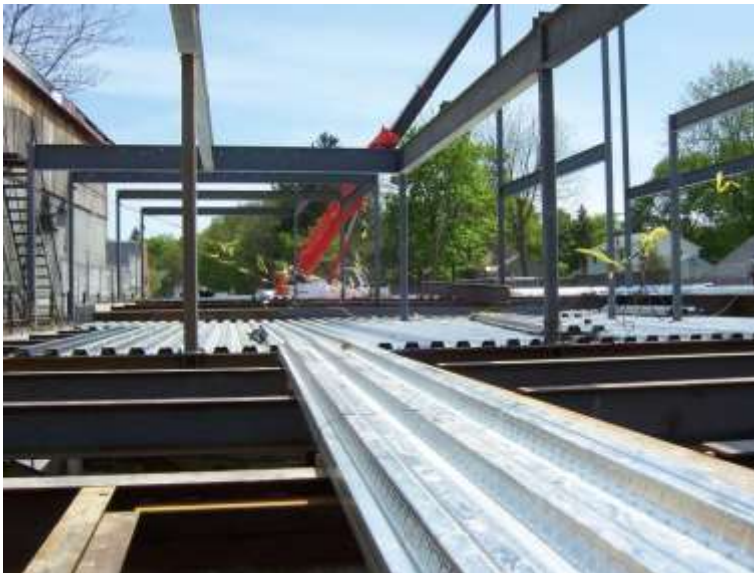
Photo #3: Steel frames support the upper floor structure
