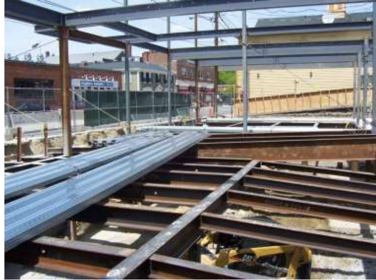
Photo #2: First floor retail space framing being installed
