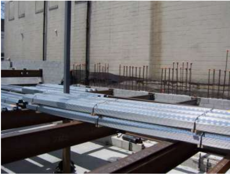
Photo #1: Composite steel deck ready for installation
