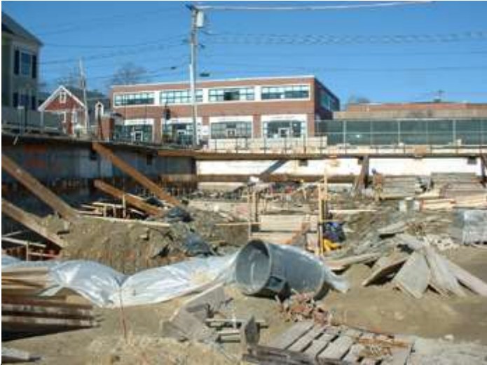
Photo #1: Braced Excavation Supports Adjacent Buildings
