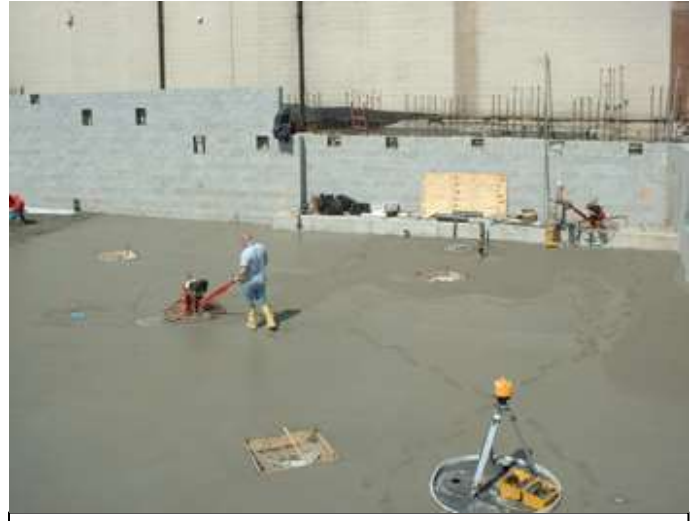
Photo #2: Underground garage concrete slab placement
