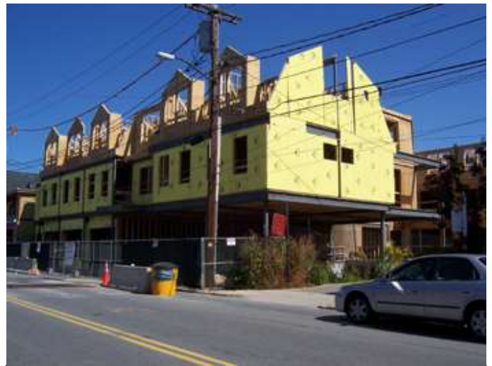
Photo #4: View of the semi finished building
