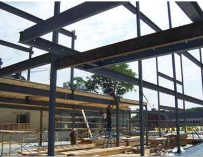
Photo #3: Steel frame with wood floors supports the upper floor structure
