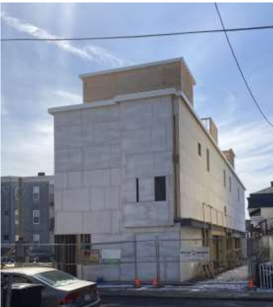
Photo #1&2: Podium Construction – View of the steel framing supporting a three story wood structure.
