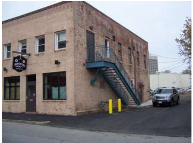
Photo #4: New exterior stair
