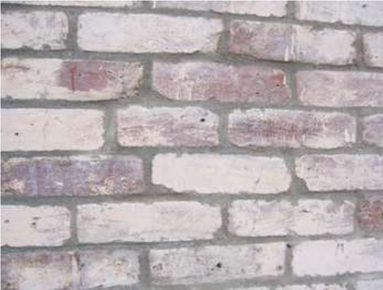
Photo #3: Repointed exterior brick wall
