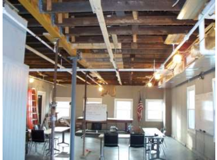
Photo #2: New LVL beam replaced existing cracked beam
