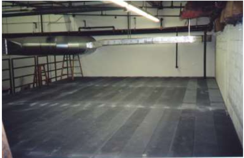
Photo #2: New Mezzanine
