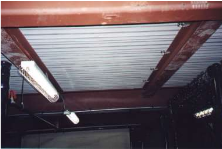
Photo #3: Steel frames for the new mezzanine
