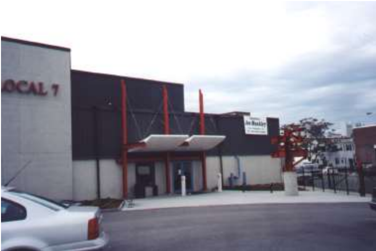
Photo #1: Building exterior canopy
