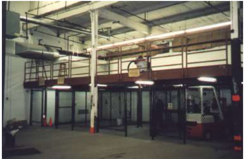
Photo #4: New Mezzanine
